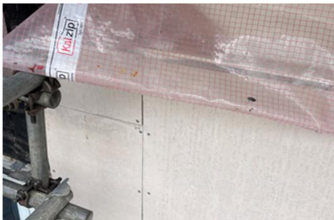
A photo showing Phase 1 South Elevation – New Versaroc sheathing board installation progressing
